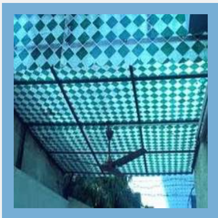
Fiber Roofing Sheets
